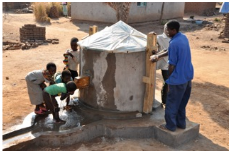
Figure 10: Photograph of the Abakus Pump with Protection
