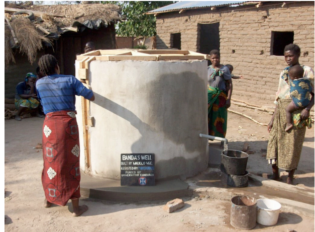
Figure 19: Photograph of the Abakus Pump built entirely by the community
