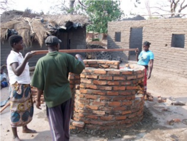
Figure 18: Photograph of the water team training women community members how to construct the Abakus Pump
