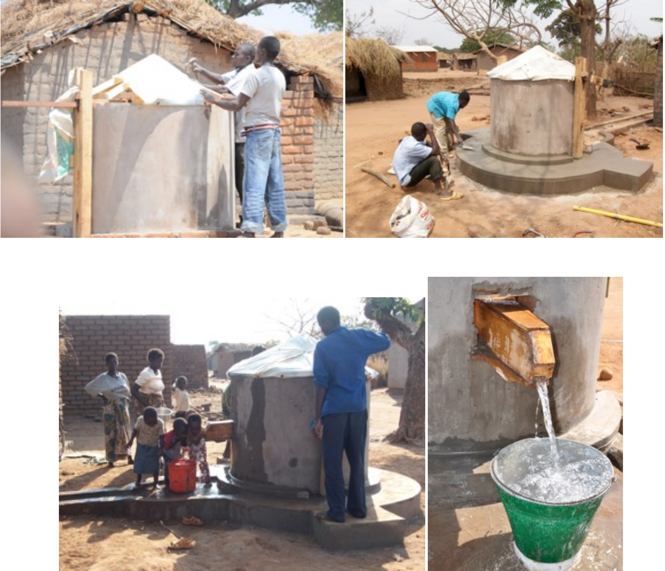
Figure 17: Photographs of the water team constructing the Abakus Pump
